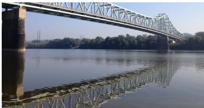
Sewickley Bridge as seen from Riverfront Park
