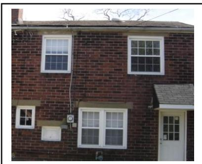
Replacement windows, door, restored coal chute, and stoop roof. Note the lintels above windows are not painted.
