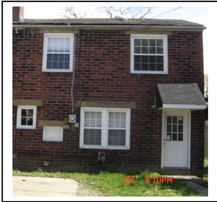
This is a good example of the window sizes, and pane configuration. Note that the lintels above the windows are not painted.
